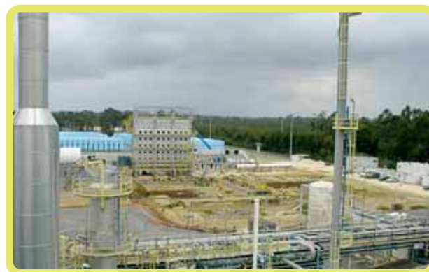
Current situation of construction works of new HyCO 3 unit
