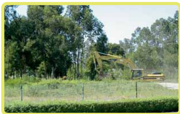
Beginning of construction works of new HyCO 3 unit
